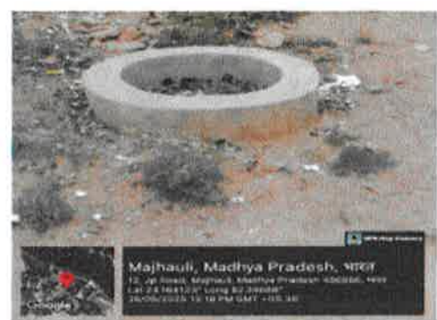
Rain Water Harvesting Pit-05
