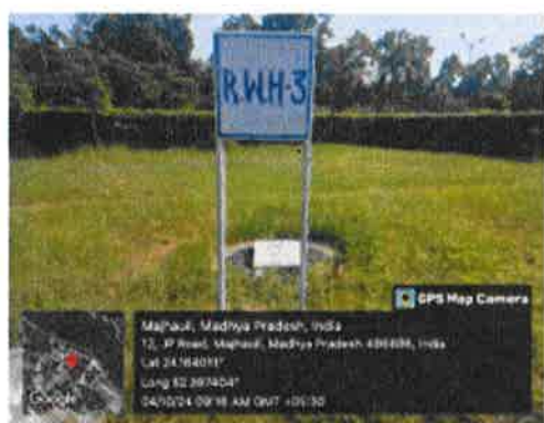
Rain Water Harvesting Pit-03
