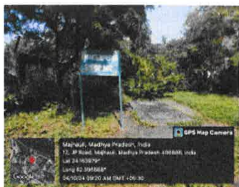
Rain Water Harvesting Pit-01
