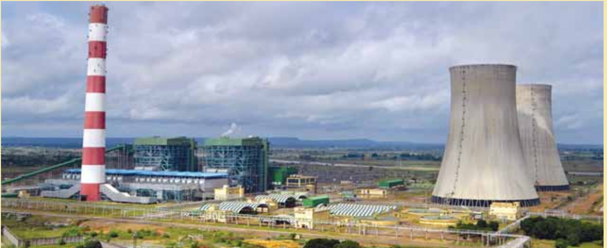
1320 MW Jaypee Nigrie Super Thermal Power Project, Nigrie, Madhya Pradesh (In Operation)
