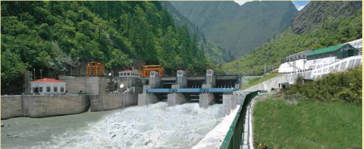
400 MW Vishnuprayag Dam, Uttarakhand (In Operation)
